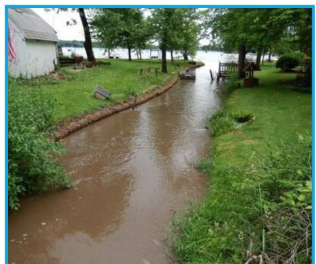
Siltation After Heavy Rains in Mason Creek Flowing into North Lake
